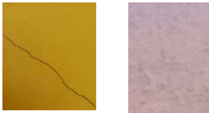
(a) (b) Gambar 1: crack (a) dan non crack (b).
